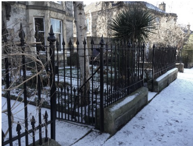
Replacement cast iron railings in Queen's Crescent, made to the original design, with low stone wall and view through gardens.
